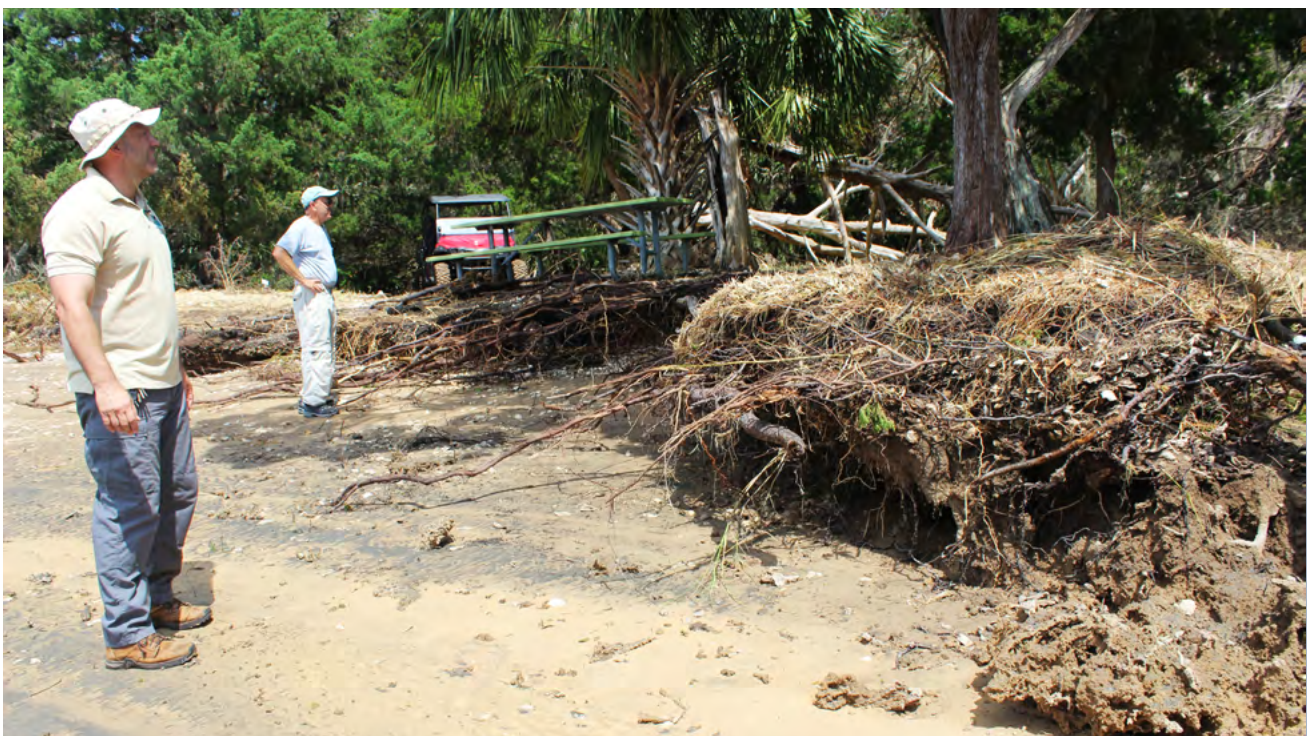
Staff from the GTM Research Reserve assess damage to Shell Bluff Landing.
